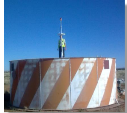
Upington, South Africa – ATNS Airport Authority ADF Antenna Installation
